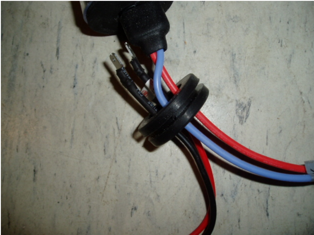
Close up of the power wires that feed the ballast which you will need to take out.
